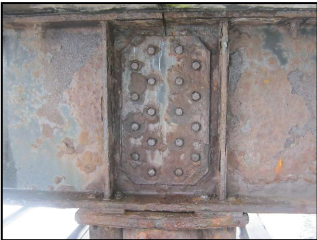
Corroded Steelwork
