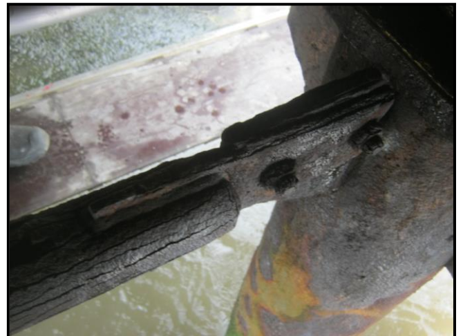
Corroded Steelwork
