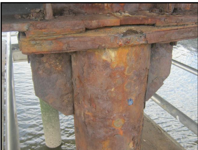
Corroded Steelwork
